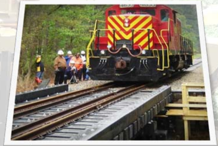
World's 1 st Plastic Railroad Bridges 12 ft max. span 120 ft total length
