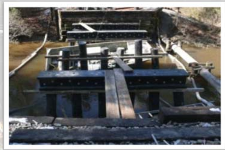
Pile Cap Installation
